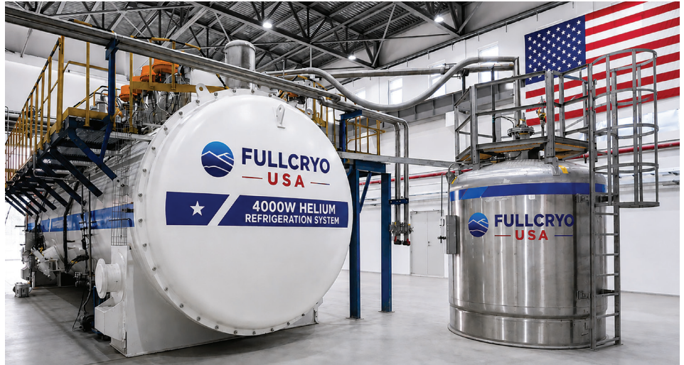
A 4,000 W x 4.5 K Helium Refrigeration unit. Credit: Fullcryo USA
